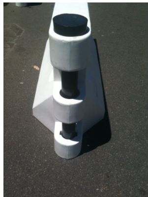
LINK PIN IN POSITION
